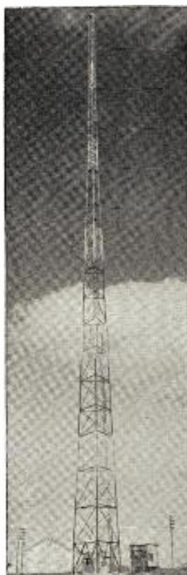
KAA-284, Owatonna, Minnesota, Northern Natural Gas Company. Truscon Self-Supporting Tower, 260 feet high.
