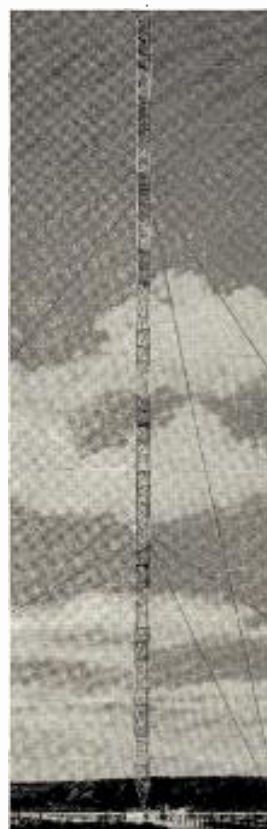
WHDH, Boston, Mass. Three Truscon Guyed Towers; 565 feet, 605 feet, and 645 feet high.
